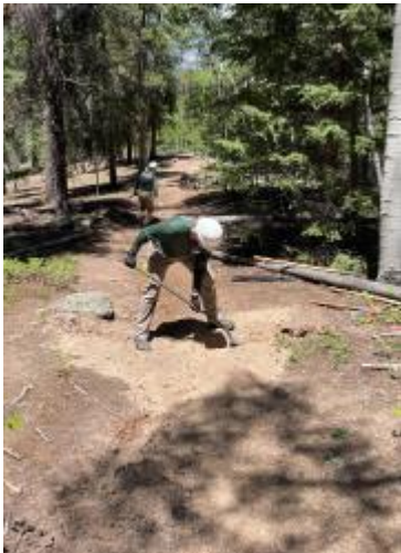
Drain Dip Water Diversion
